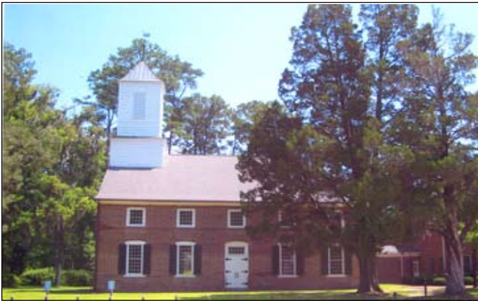
Jerusalem Evangelical Lutheran Church in Georgia, across the river from the site of Purrysburg, was completed in 1769. Inside its twenty-one-inch walls, services are still held every Sunday. Photo by Lyman Wooster.
